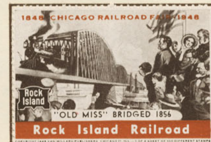
A mighty web-like mass of wood superstructure resting on stone piers which took the river in 250-foot leaps was the first bridge built by man to cross the Mississippi River, completed in 1856.
