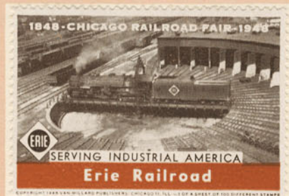
A powerful Series 3300 Erie Railroad locomotive completely spans the turntable of a roundhouse where it receives periodic maintenance.
