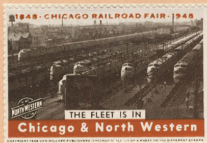
North Western with its great fleet of Diesel-powered Streamliners has a very modern Diesel servicing and repair plant at the railroad's Chicago shops costing well over $1,000,000.
