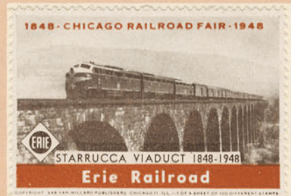
Starrucca Viaduct, 100 years old, carries the heavy traffic on the Erie Railroad's main line across a valley near Susquehanna, Penna.
