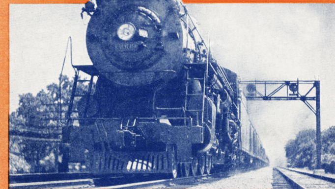
One of the Burlington's great steam trains
