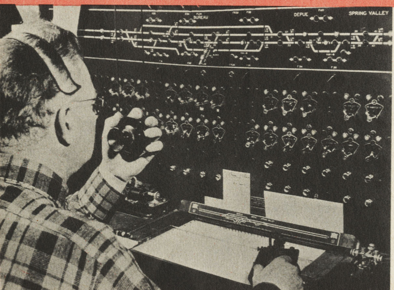
TRAFFIC CONTROL —This is the Centralized Traffic Control console . . . its control alert operator knows the position of every train in his area. He sets the signals and is in constant touch with way stations by telegraph and telephone, talks directly with radio-equipped trains. Result—greater safety, faster train movements, in larger volume.
