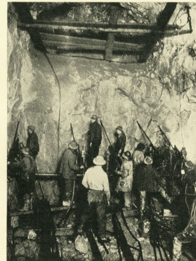
Drilling on last barrier in main bore.
