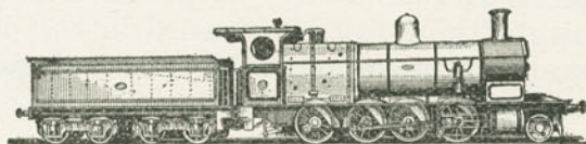
Consolidation Freight or Goods Locomotive, New South Wales. Diameter of cylinders, 21 inches; stroke, 26 inches.
