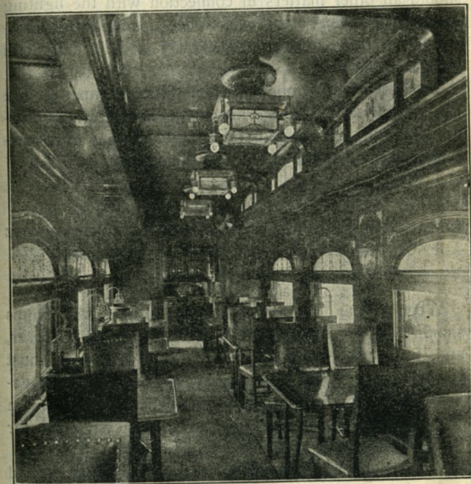
FIG. 58. INVERTED BURNER LAMPS IN DINING CAR.
