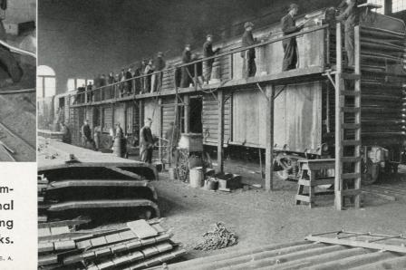
*Right:* In this picture, nearly completed box cars are receiving final touches to their roofs prior to being moved out on the yard tracks.
