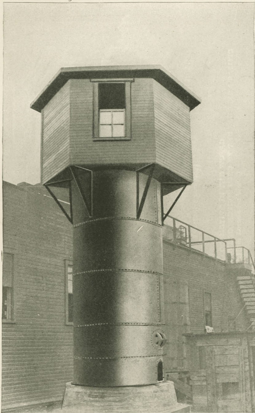
TYPE OF KENNICOTT WATER SOFTENER USED ON THE SOUTHERN PACIFIC AND BIG FOUR RAILWAYS (Kennicott Water Softener Co.)
