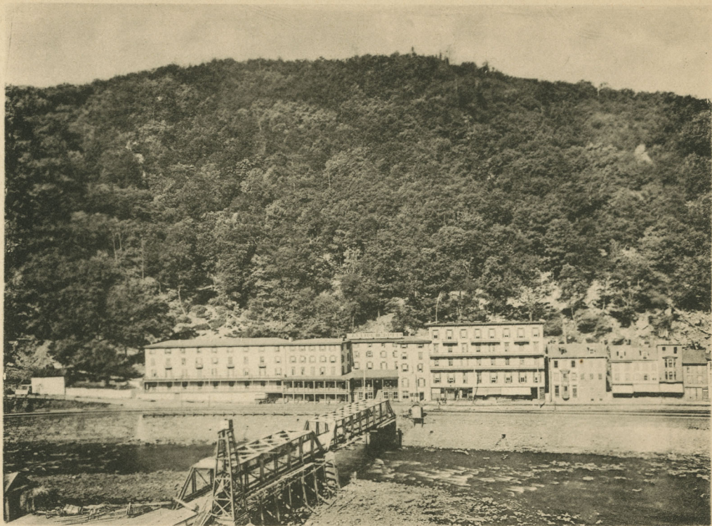
MANSION HOUSE AND SOUTH MOUNTAIN
